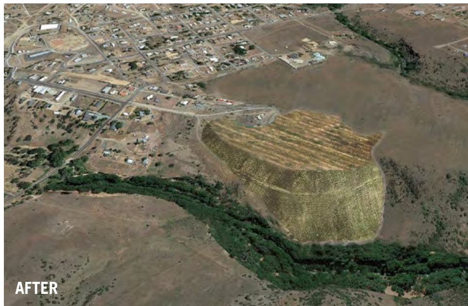
Figure 16B. Completed waste repository at the former Humboldt Smelter property.
