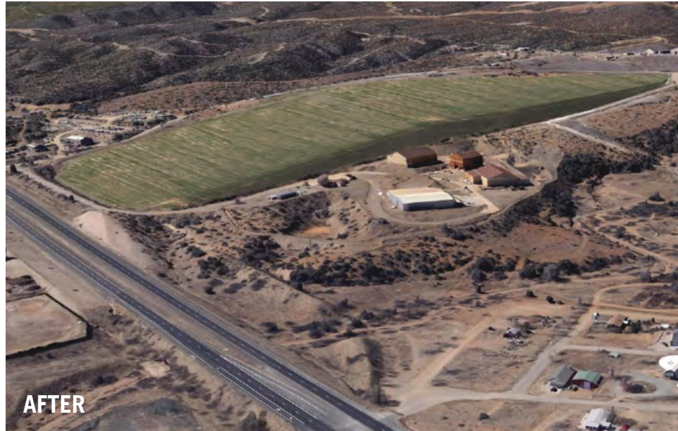
Figure 15B. Regraded and revegetated waste repository at the former Iron King Mine tailings pile after cleanup
