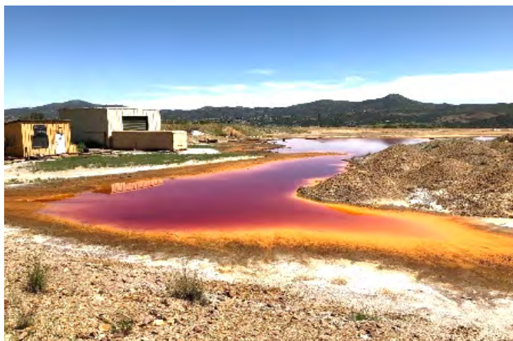
Stormwater retention basin on the lower tier of the mine tailings pile.
